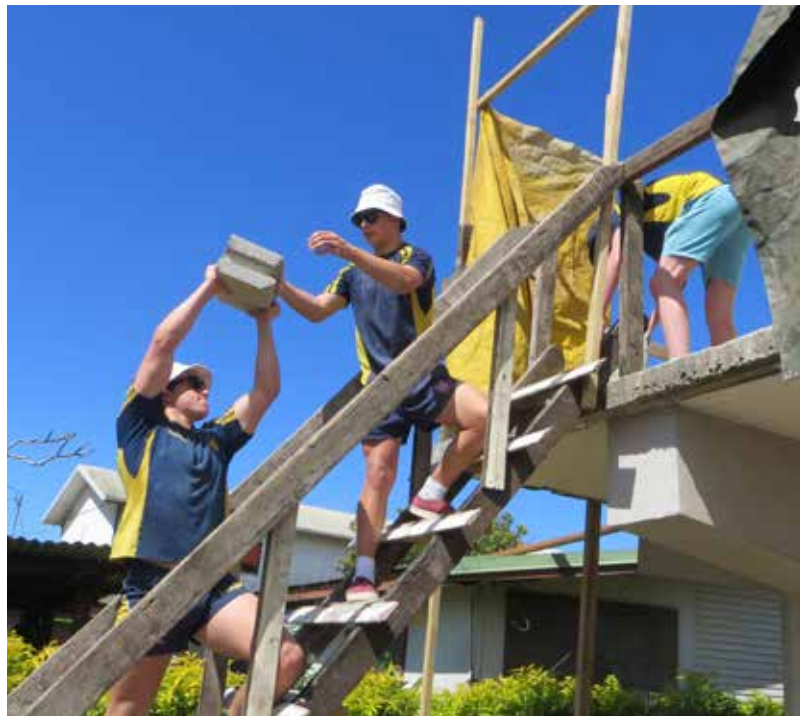
The construction of new Sunday School building at Paton Memorial Church begins in October 2015.
