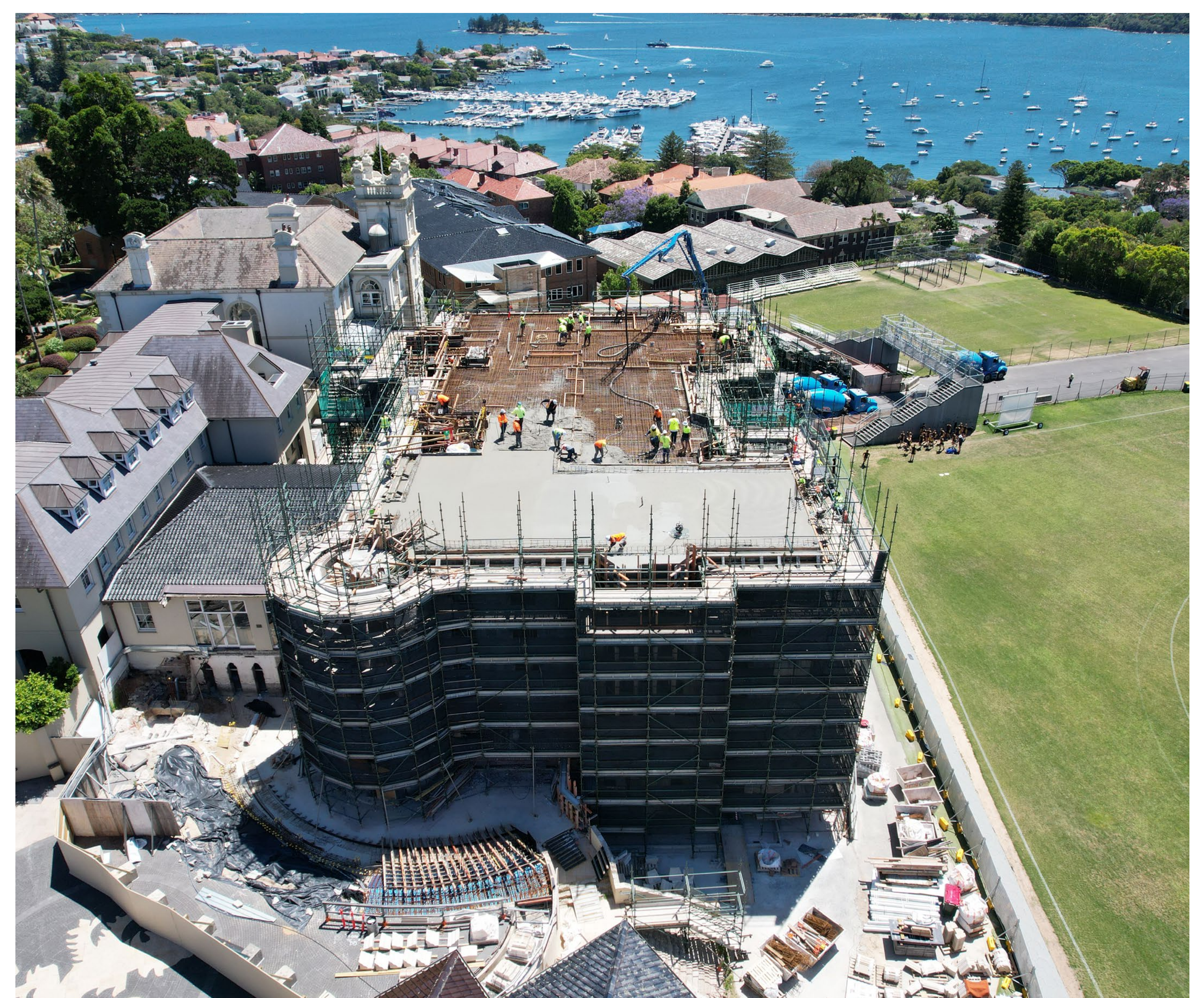
Work underway Feb 2023
