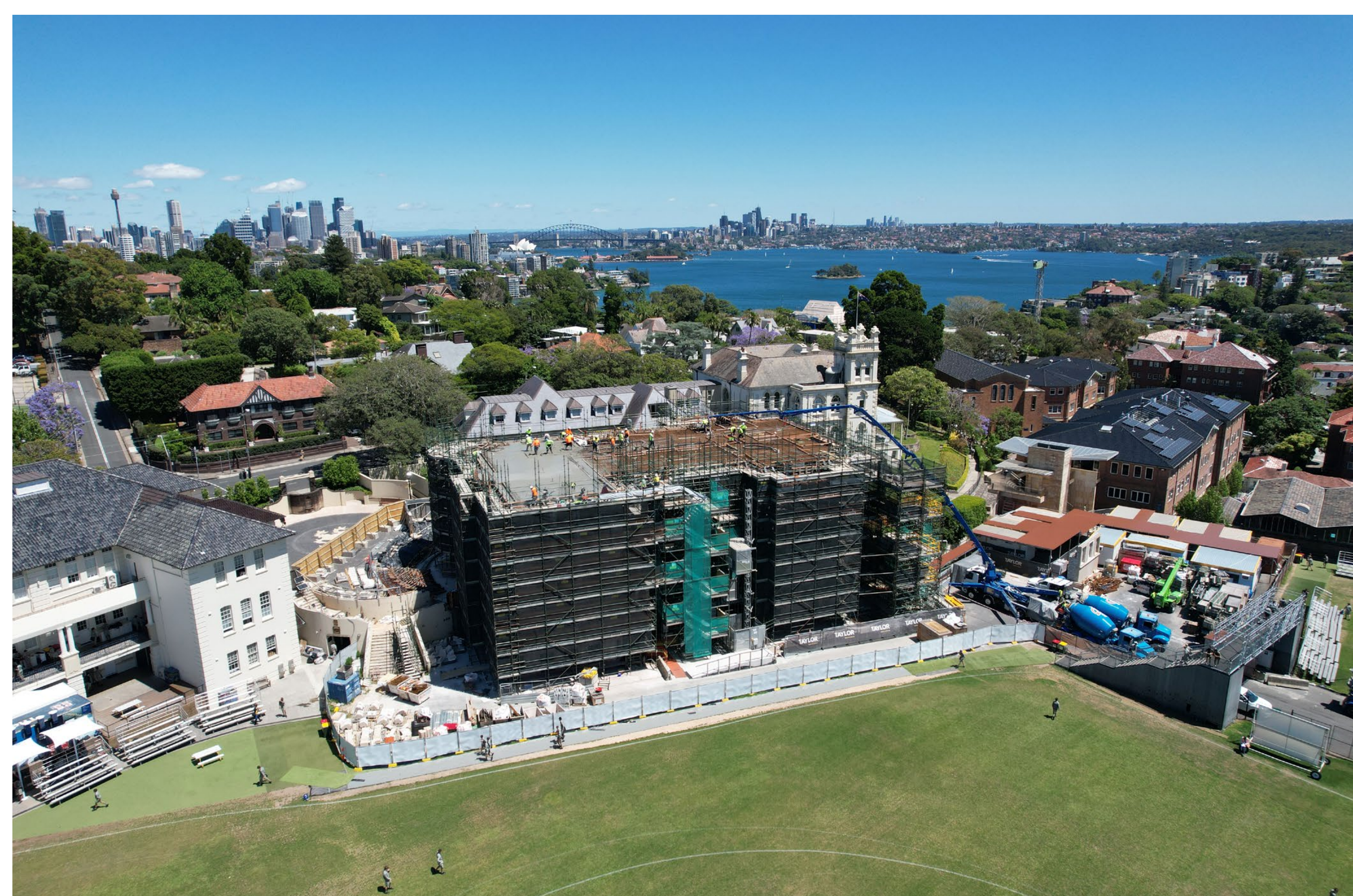
Work underway Feb 2023
